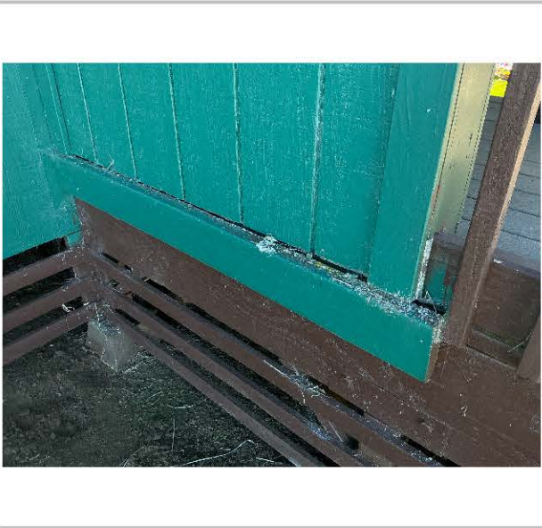
Polipoli-Spring-State-Recreation-Area_Cabin-Structural Repairs and Painting_Remove and Replace Rotted Boards and T&G Siding
