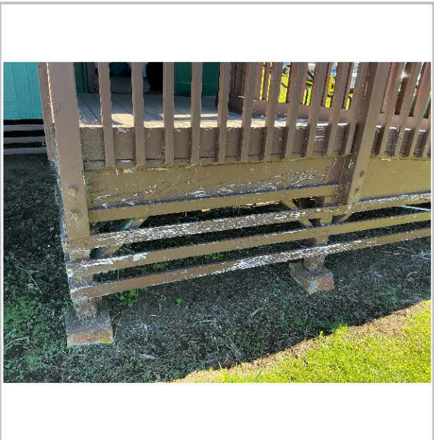
Polipoli-Spring-State-Recreation-Area_Cabin-Structural Repairs and Painting_Remove and Replace Rotted Boards and T&G Siding
