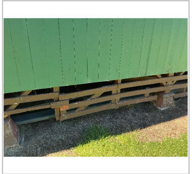
Polipoli-Spring-State-Recreation-Area_Cabin-Structural Repairs and Painting_Remove and Replace Rotted Post
